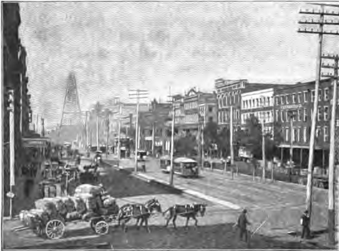
Canal Street, New Orleans.
